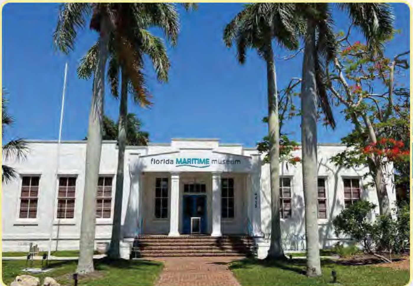
Cortez Rural Schoolhouse , photo by Tori Chasey, Photo courtesy of Historical Resources
