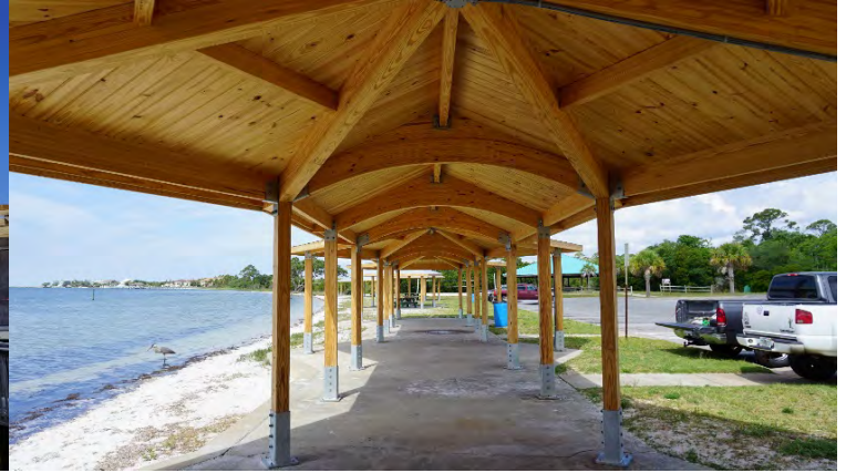
Recreation Department Gazebo project substantially complete
