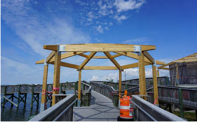
Recreation Department Gazebo project in-progress
