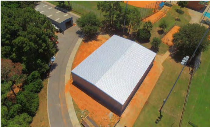
Recreation Department multi-purpose building
