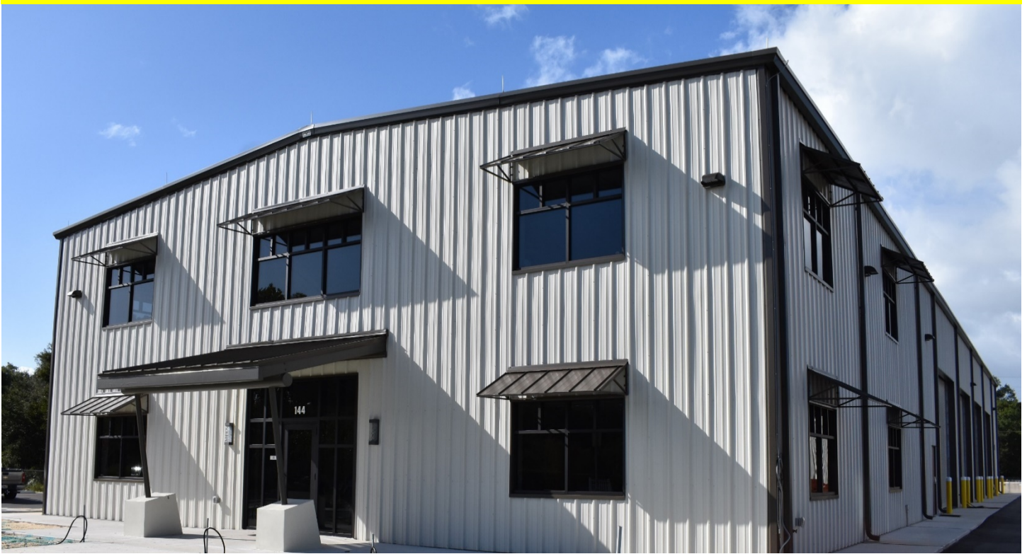
Public Works Utility Building Completed Summer 2019
