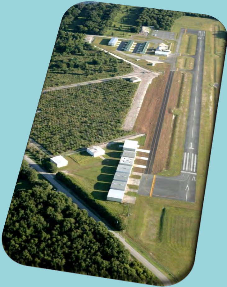
Umatilla Airport Project: Completion of Parallel Taxiway
