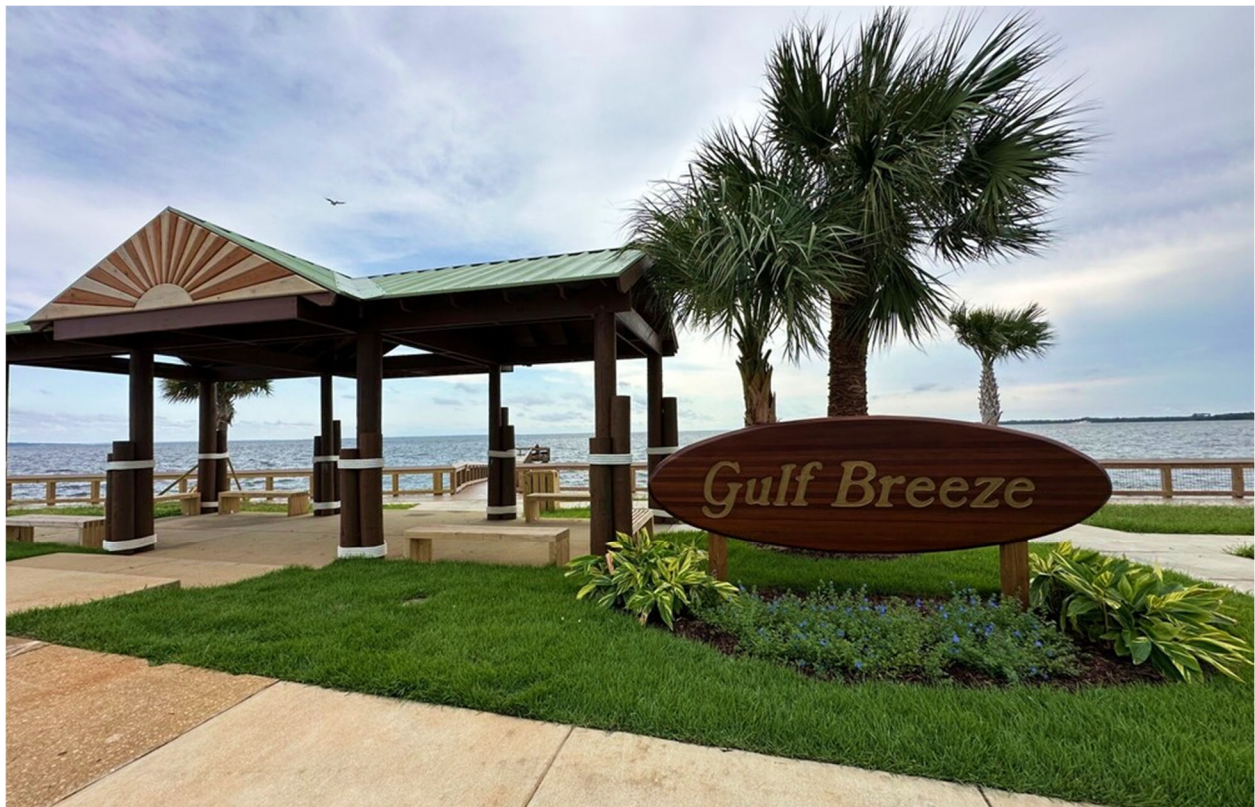
Fishing Pier at Mariners Landing
