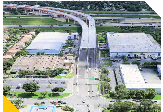
Project 87410 – SR 874 Ramp Connector to SW 128th Street
