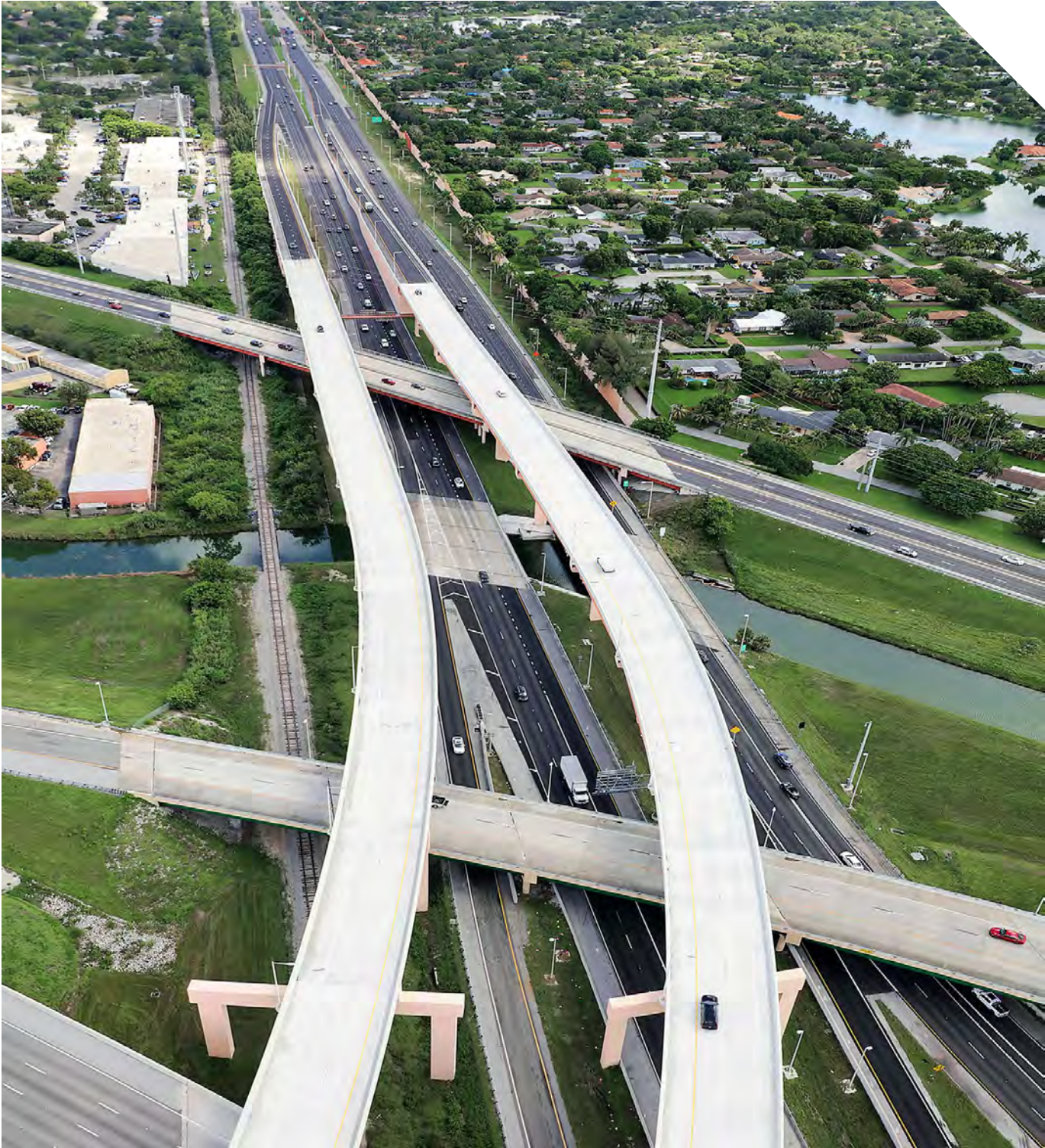
New Bridge approach to southbound SR 874.
