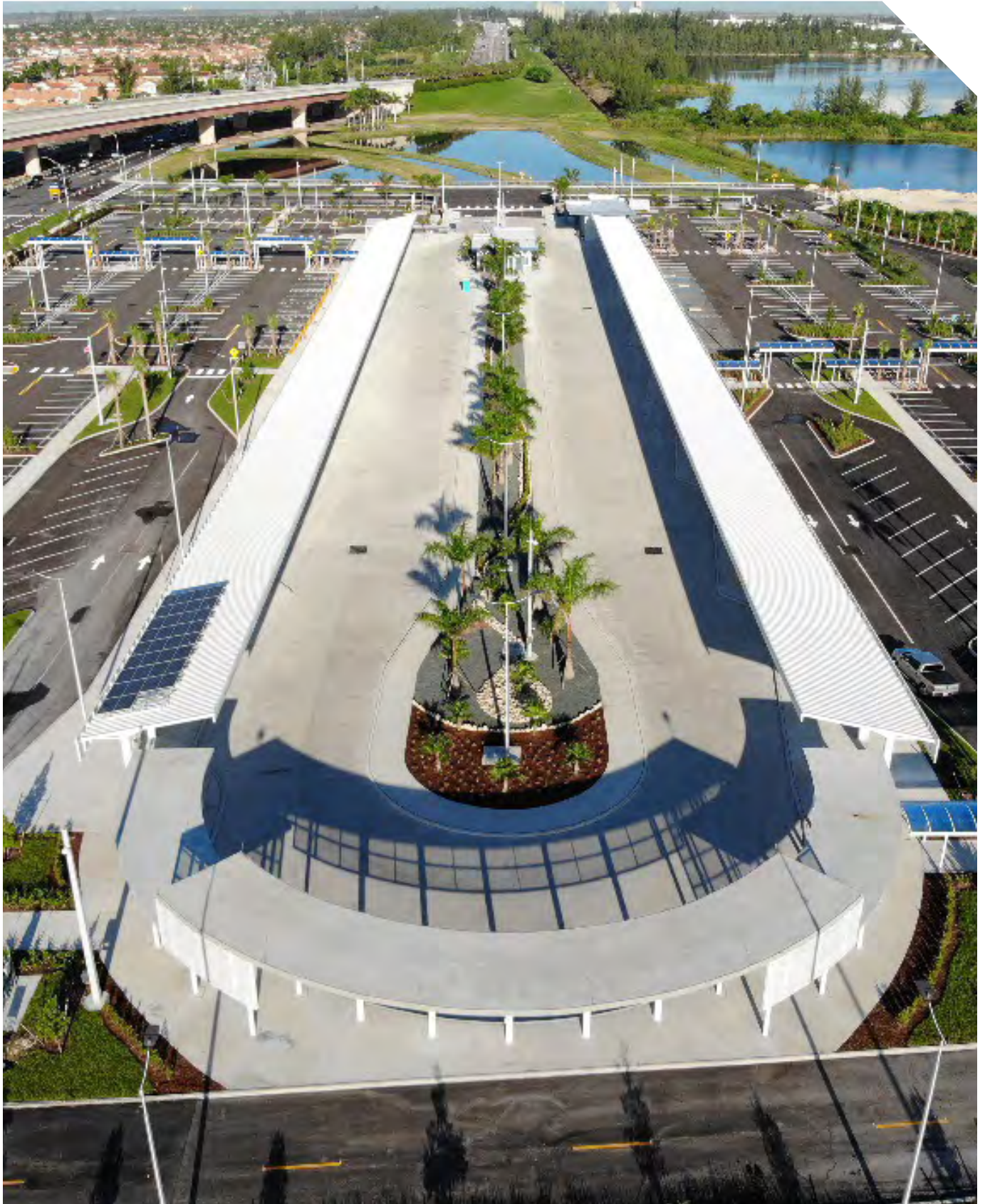
The Dolphin Station Park and Ride Transit Facility.
