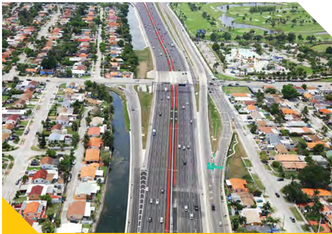
Project 83628 – SR 836 Operational, Capacity and Interchange Improvements
