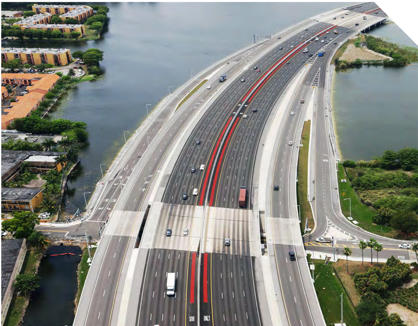
SR 836 Operational, Capacity, and Interchange Improvements looking westbound at NW 45th Avenue.
