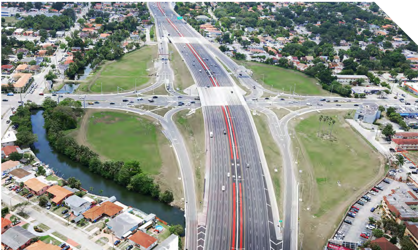
SR 836 Operational, Capacity and Interchange Improvements, looking westbound on SR 836 approaching NW 27th Avenue.
