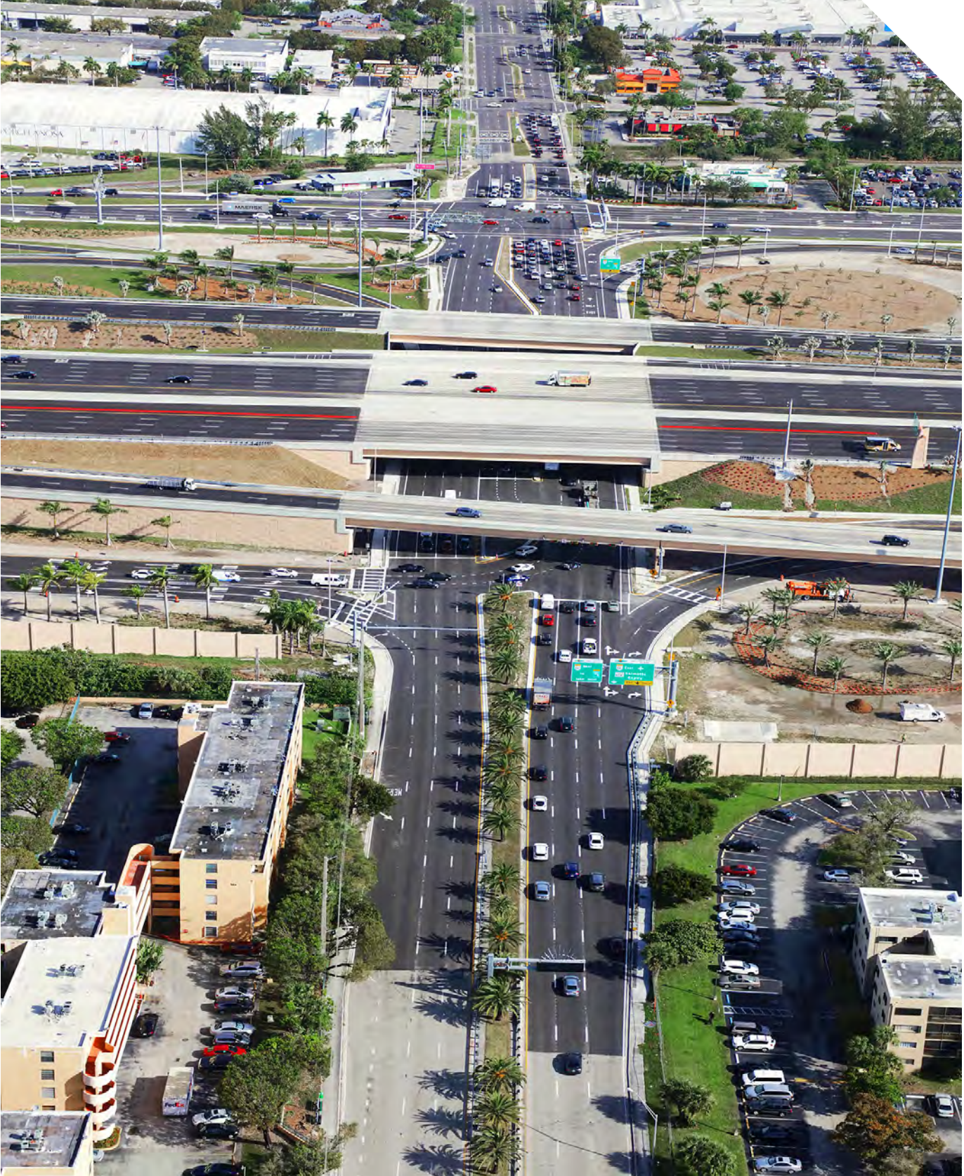
SR 836 Interchange Modifications at 87th Avenue, looking northbound at 87th Avenue.
