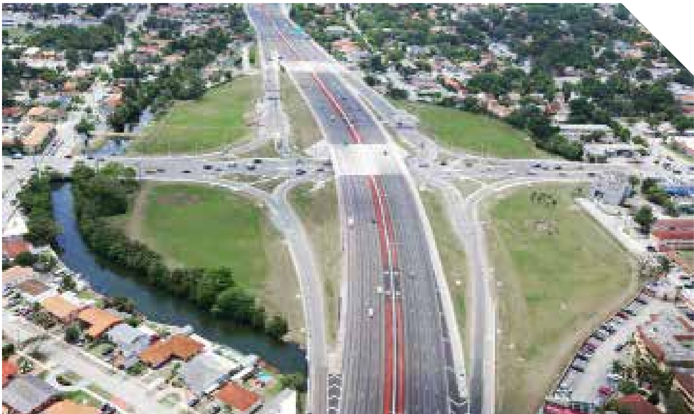
SR 836 Operational, Capacity and Interchange Improvements, looking westbound on SR 836 approaching NW 27th Avenue.
