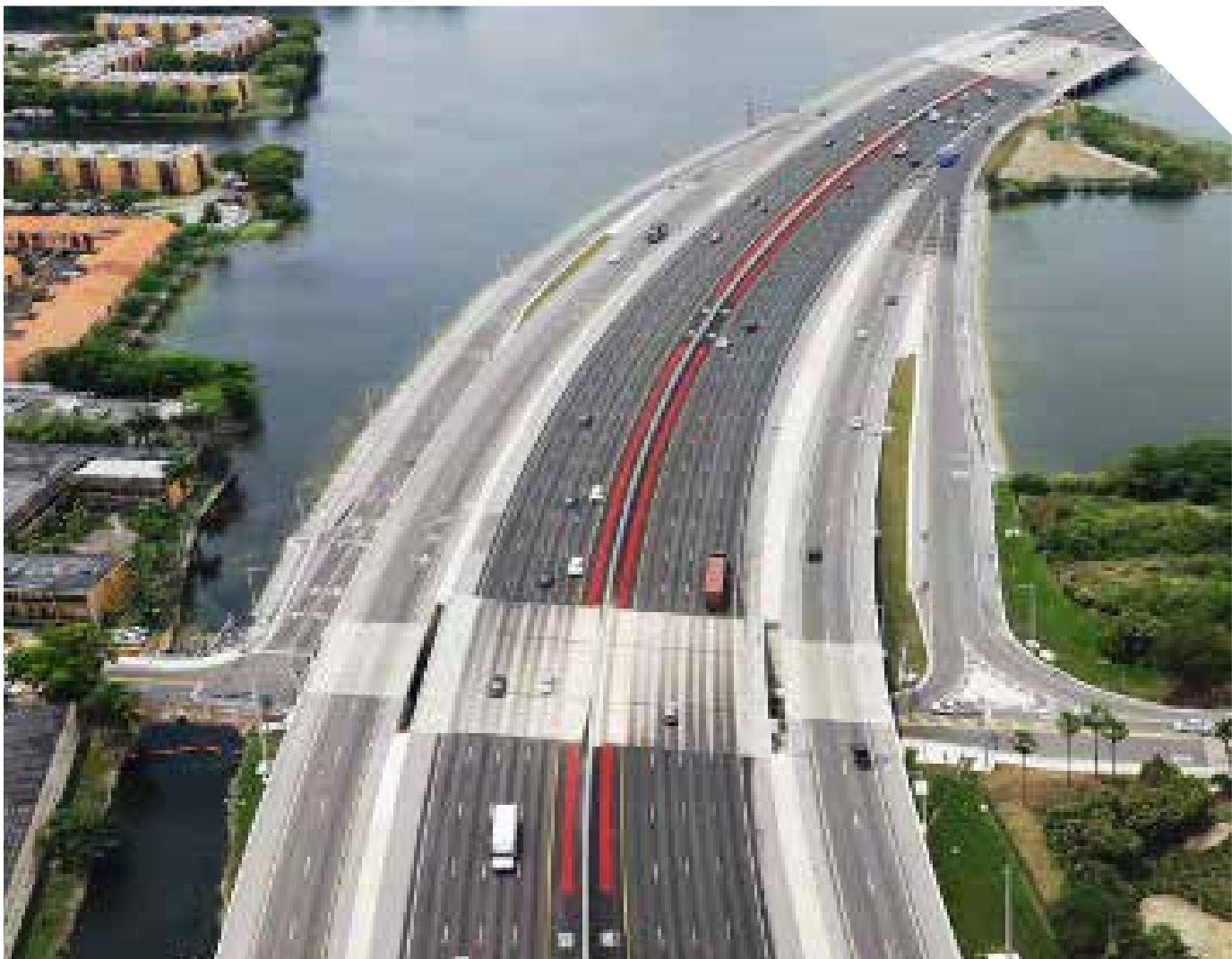
SR 836 Operational, Capacity, and Interchange Improvements looking westbound at NW 45th Avenue.
