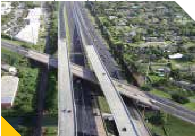
Project 87410 – SR 874 Ramp Connector to SW 128th Street
