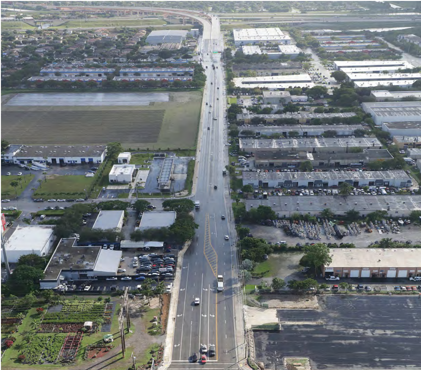
SW 128th Street at SW 122nd Avenue looking toward SR 876 Ramp Connector.
