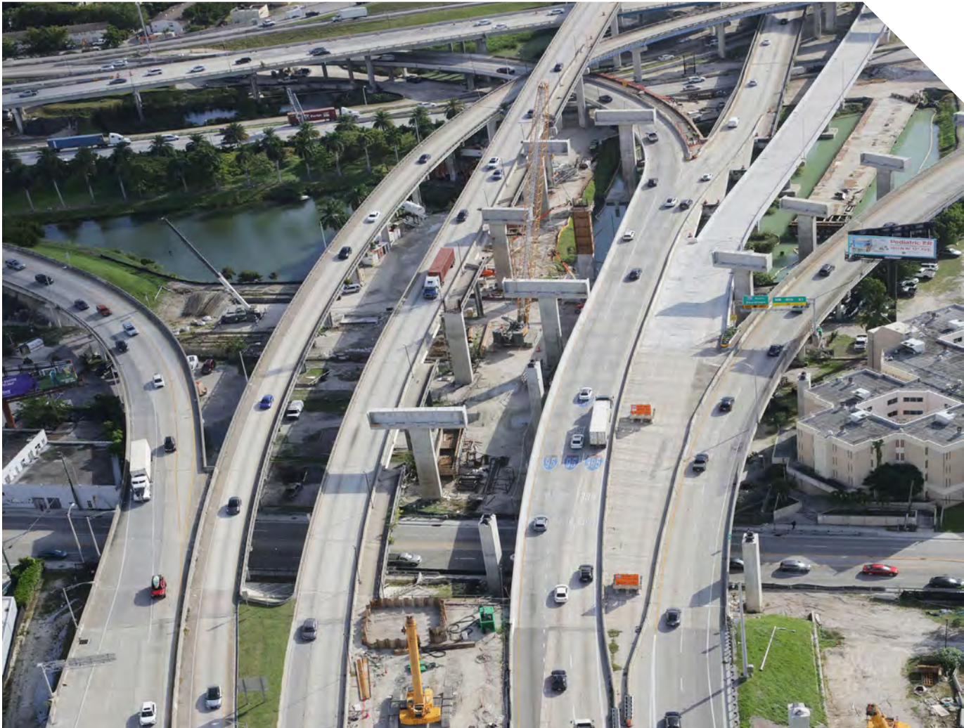
The I-395 Bridge Project.
