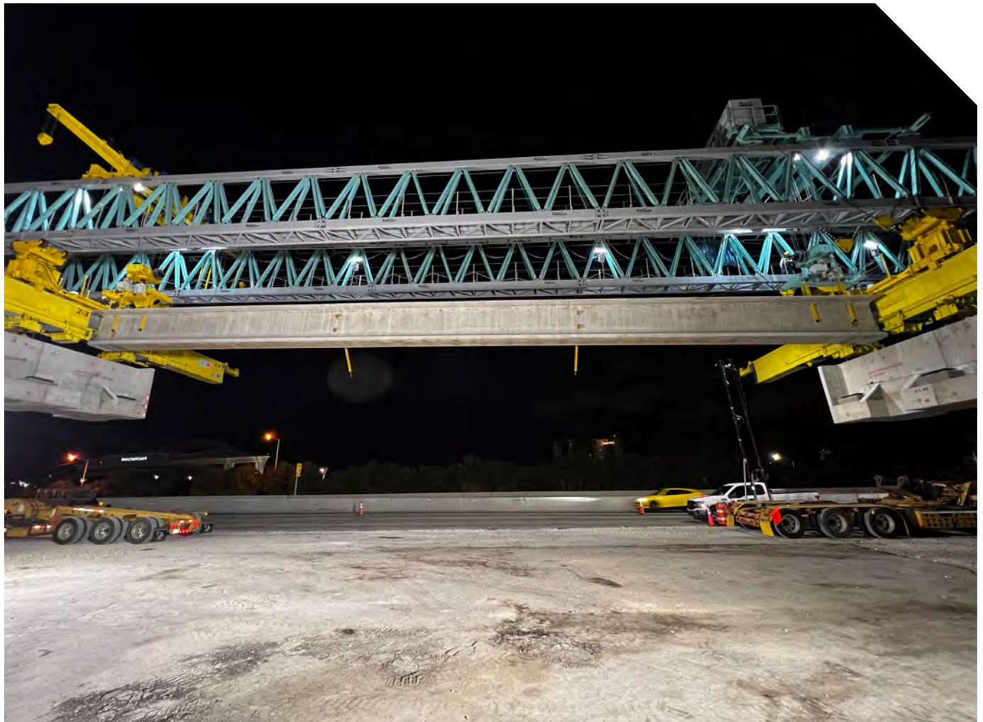
Beam setting activities.
