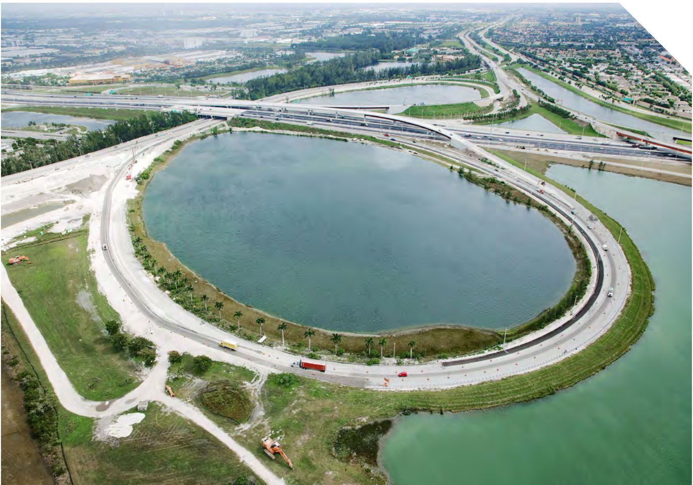
SR 836 new HEFT ramp extensions.
