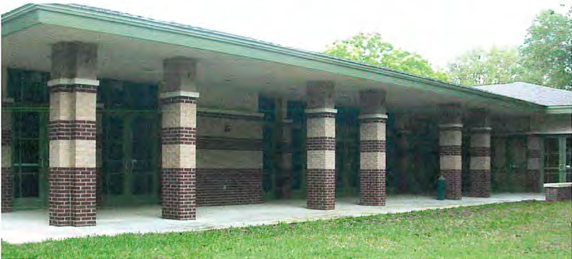
Covered patio outside multi-media room on north side
