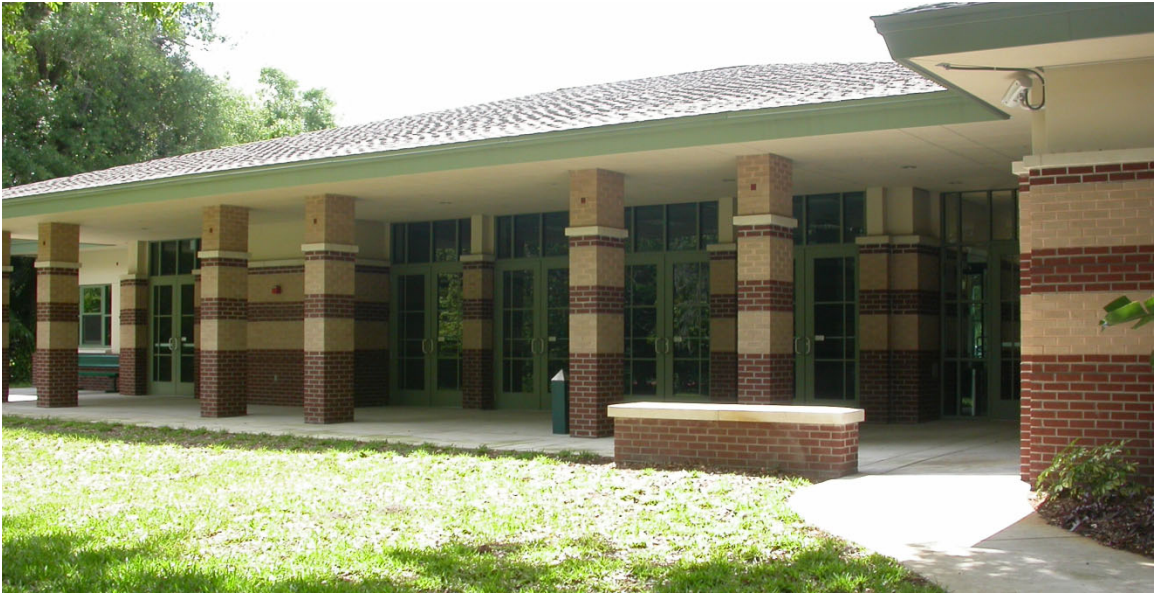
Recreation Center, south elevation from the tennis courts
