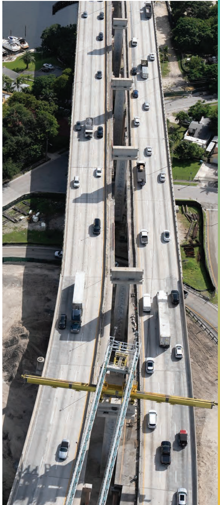
SR 836 double-decker over the Miami River under construction
