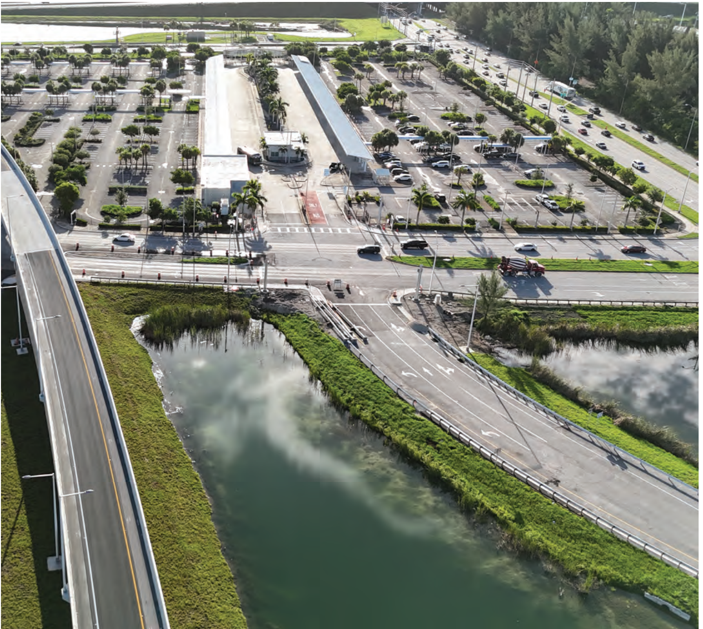
New access ramps to and from Dolphin Station Park-And-Ride looking east.
