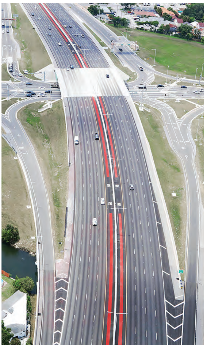
SR 836 Operational, Capacity, and Interchange Improvements looking westbound at NW 45th Avenue.
