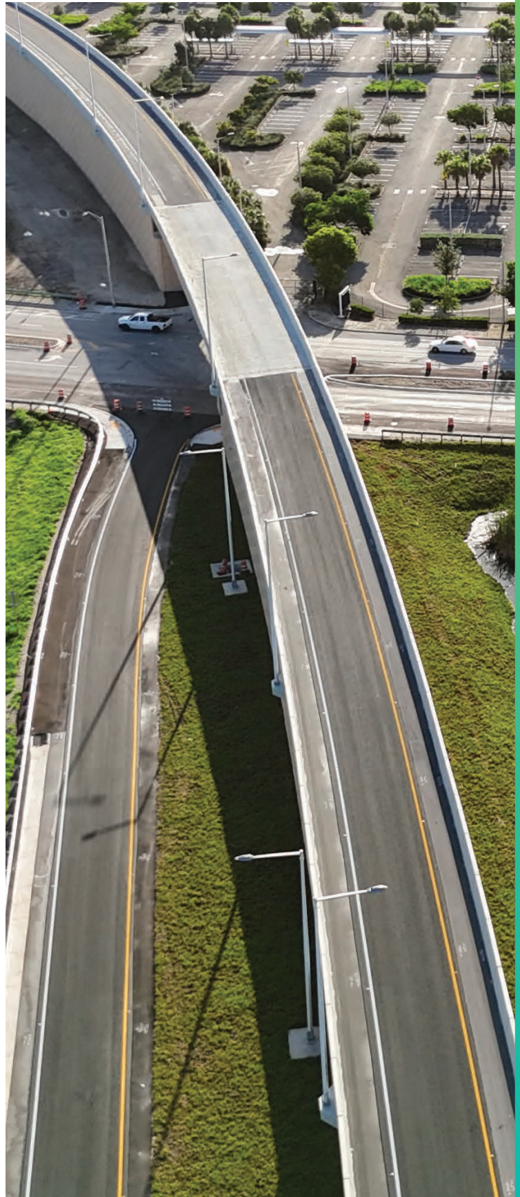
New access ramps to and from Dolphin Station Park-And-Ride looking east.
