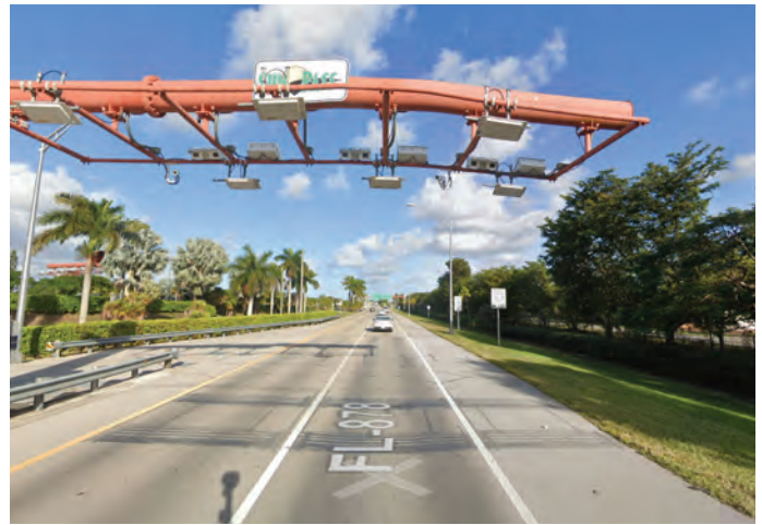
SR 878 Eastbound Ramp from SR 874
