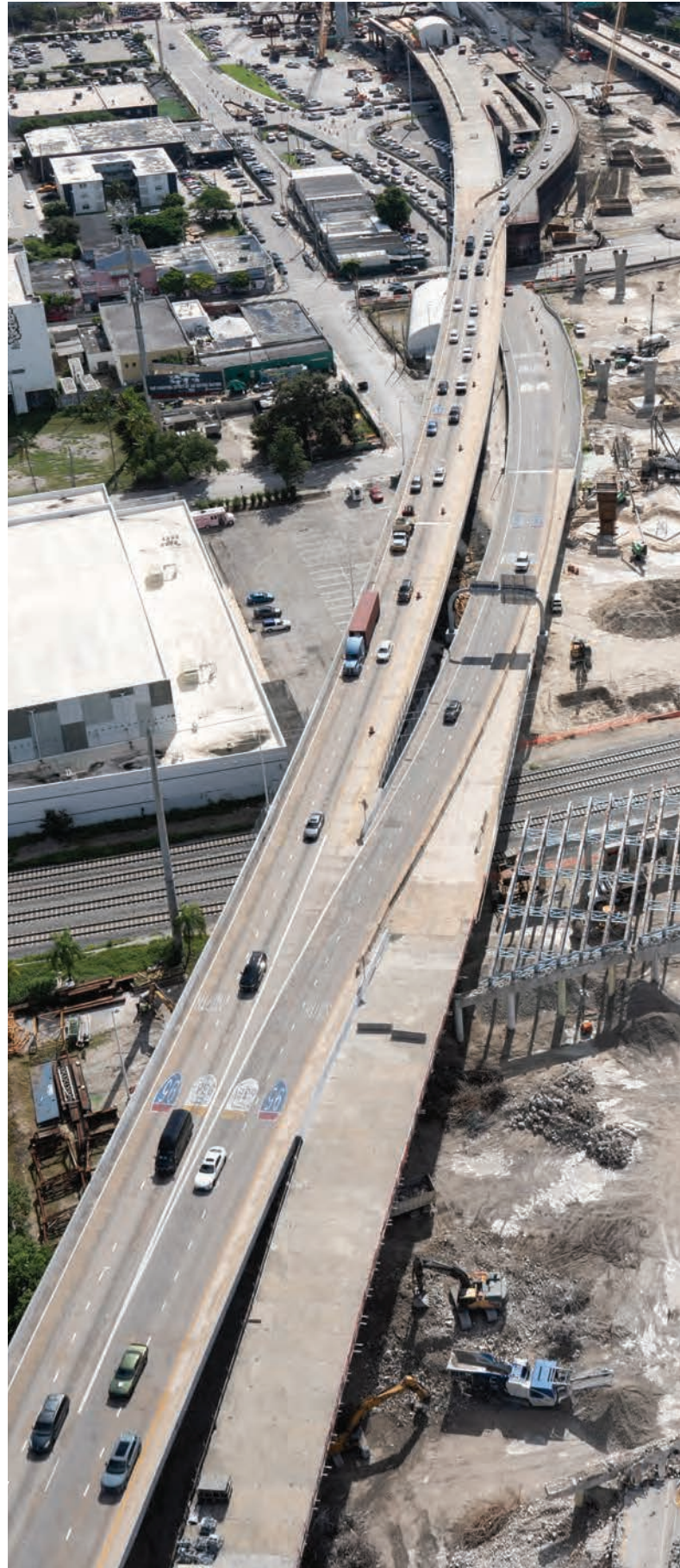
The I-395 signature bridge under construction.
