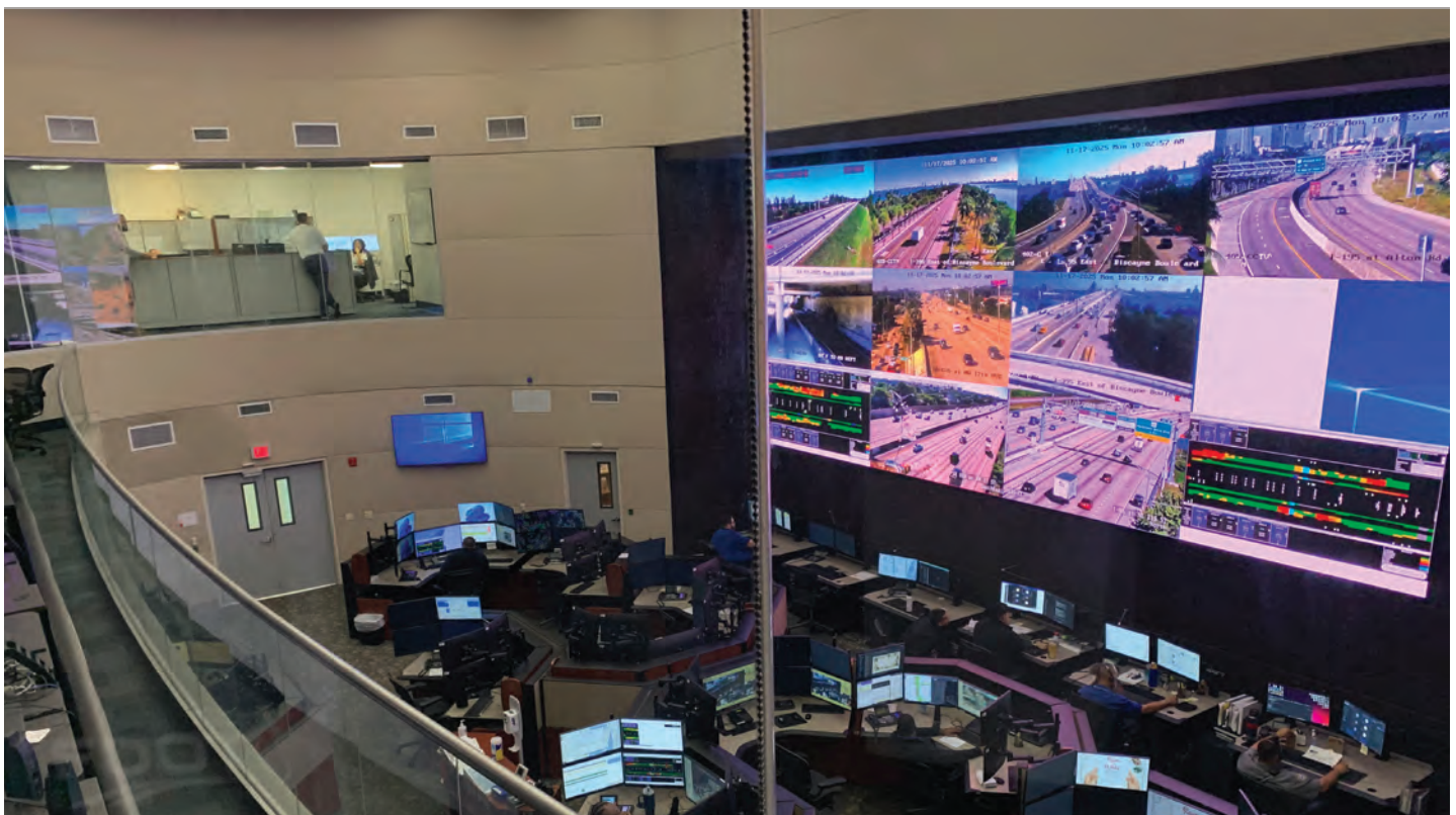
Transportation Management Center (TMC)
