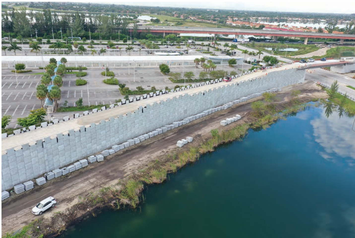
Construction of new access ramp to Telemundo Way.
