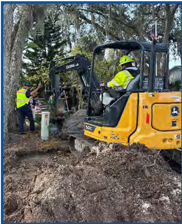
Sewer Lateral Installation
