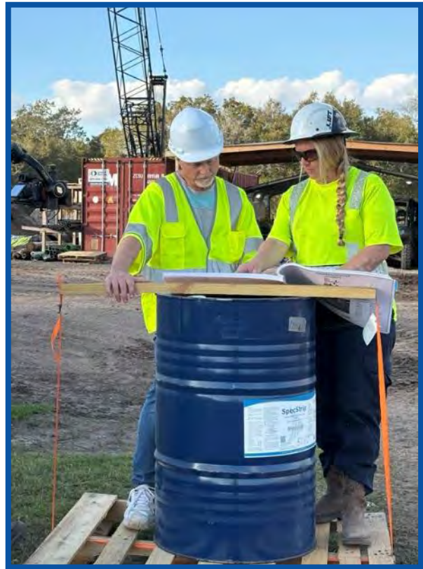
Toho employees review blueprints for expansion of South Bermuda Water Reclamation Facility
