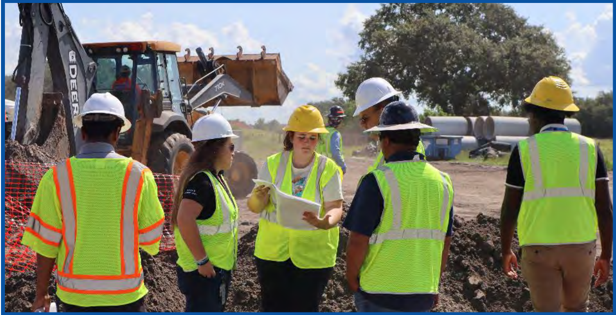
Engineering oversees Horizontal Directional Drilling Project
